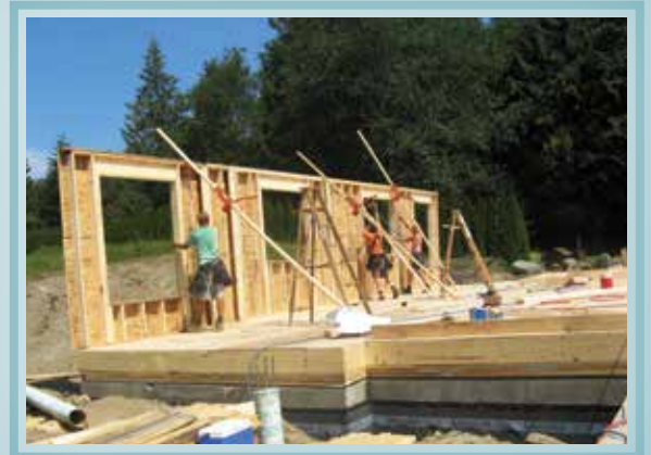
First walls going up!
